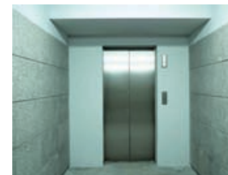
HIGH-TECH ELEVATORS WITH GENERATOR BACK-UP
